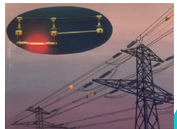
Paris Airport, FRANCE. Working since 1973!
